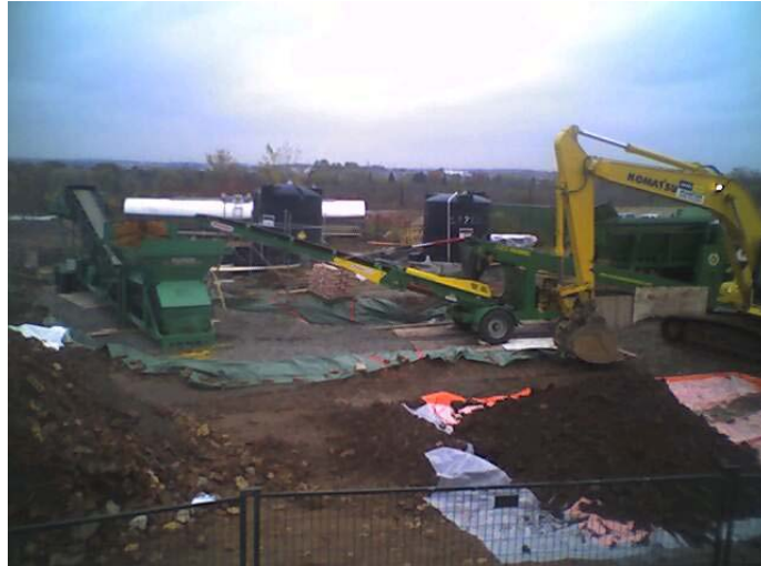
Ex-situ treatment of soils impacted with heavy metals, at hazardous levels, using OxyTek™-ADT. PHC impacted soils were also treated ex-situ, using OxyTek-L™.
