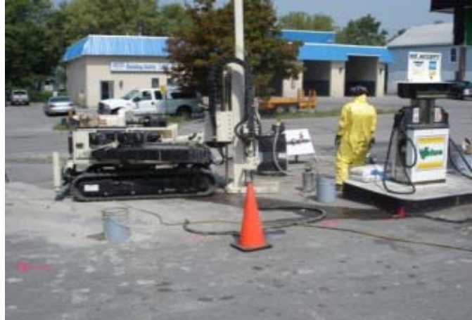
OxyTek-L™ being injected into wells as station continued to operate.
