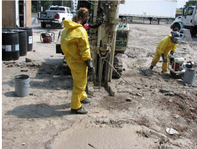
In-situ remediation with OxyTek-L™ with product being injected
