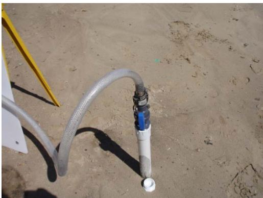
Injection well with OxyTek-L™ being loaded
