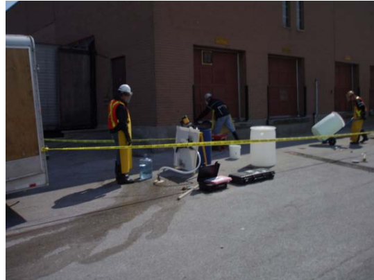
Injecting OxyTek-L™ into injection wells around building
