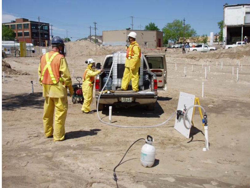
Injecting OxyTek-L™ into injection wells
