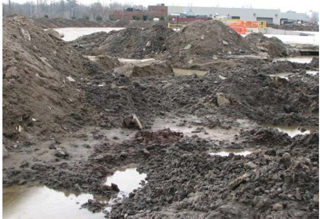
View of site during treatment of soil stockpiles.
