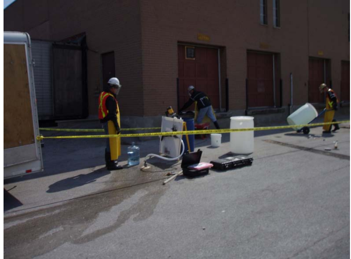
OxyTek-S™ being injected in wells installed outdoors.
