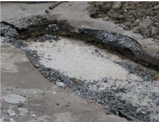
Chemical reaction of OxyTek-S™ in former tank farm area
